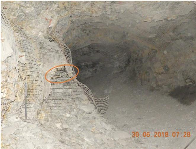
Figure 8: Area subject to seismic event with one of the Vulcan Bolts highlighted.
